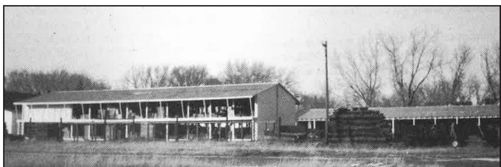
After Sandy Larsen took over the Doyle and McMillan Lumber Yard in Thedford, he tore out the old storage sheds and built new storage for lumber and supplies as this picture shows in the Pictorial History of the Sandhills . The Larsens operated the business for 40 years and in 1975 sold it to Tim and Kenneth Neal, who formed Neal Lumber Company, Inc.
